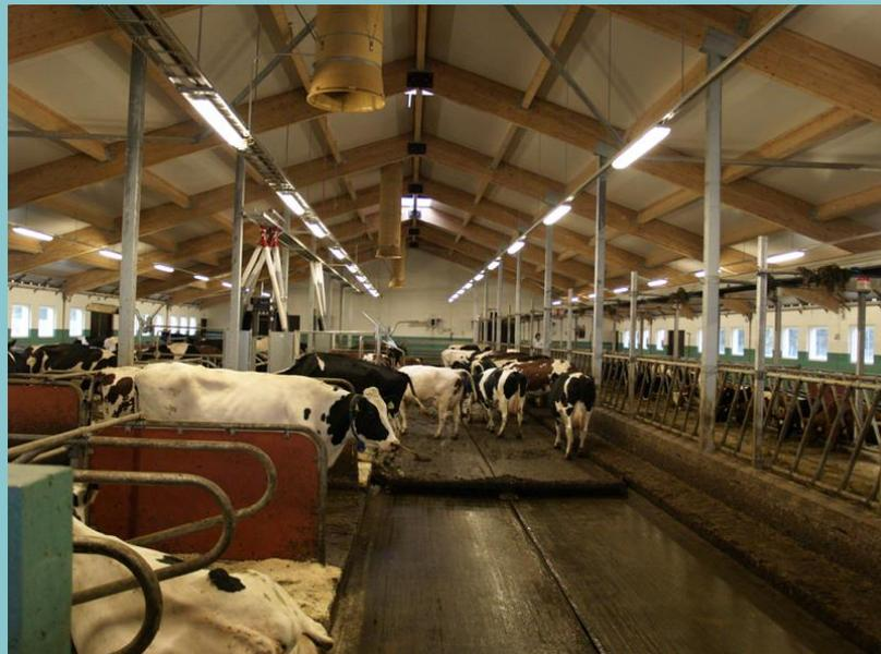
**Manure scraper in loose housing with slatted floor (rakolattia)**
